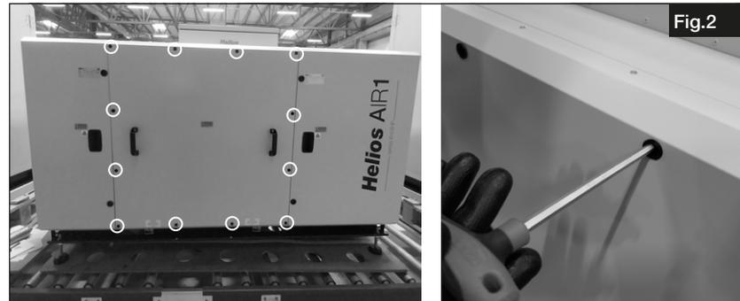
3. Remove the sheet on the bypass channel. The recirculation damper is installed here, see Fig.3.
