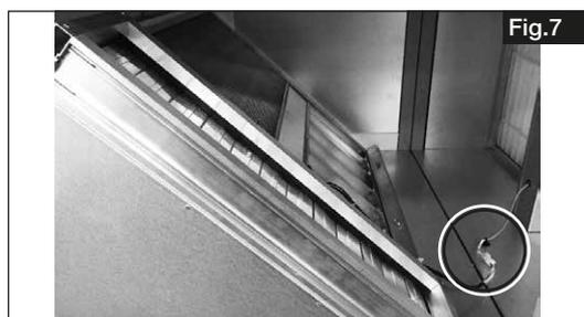
8. After installation of the recirculation damper, adjust the settings in the commissioning assistant. In this respect, observe the corresponding chapter in the installation and operating instructions for the respective AIR1 ventilation unit!
